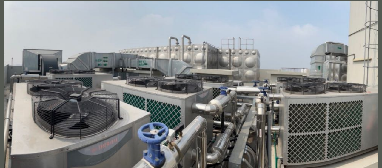
~ 500KW Heat Pump Water Heater
